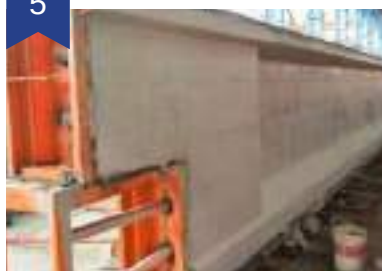
Pengecoran dan Pemadatan Beton Casting and Compaction of Concrete
